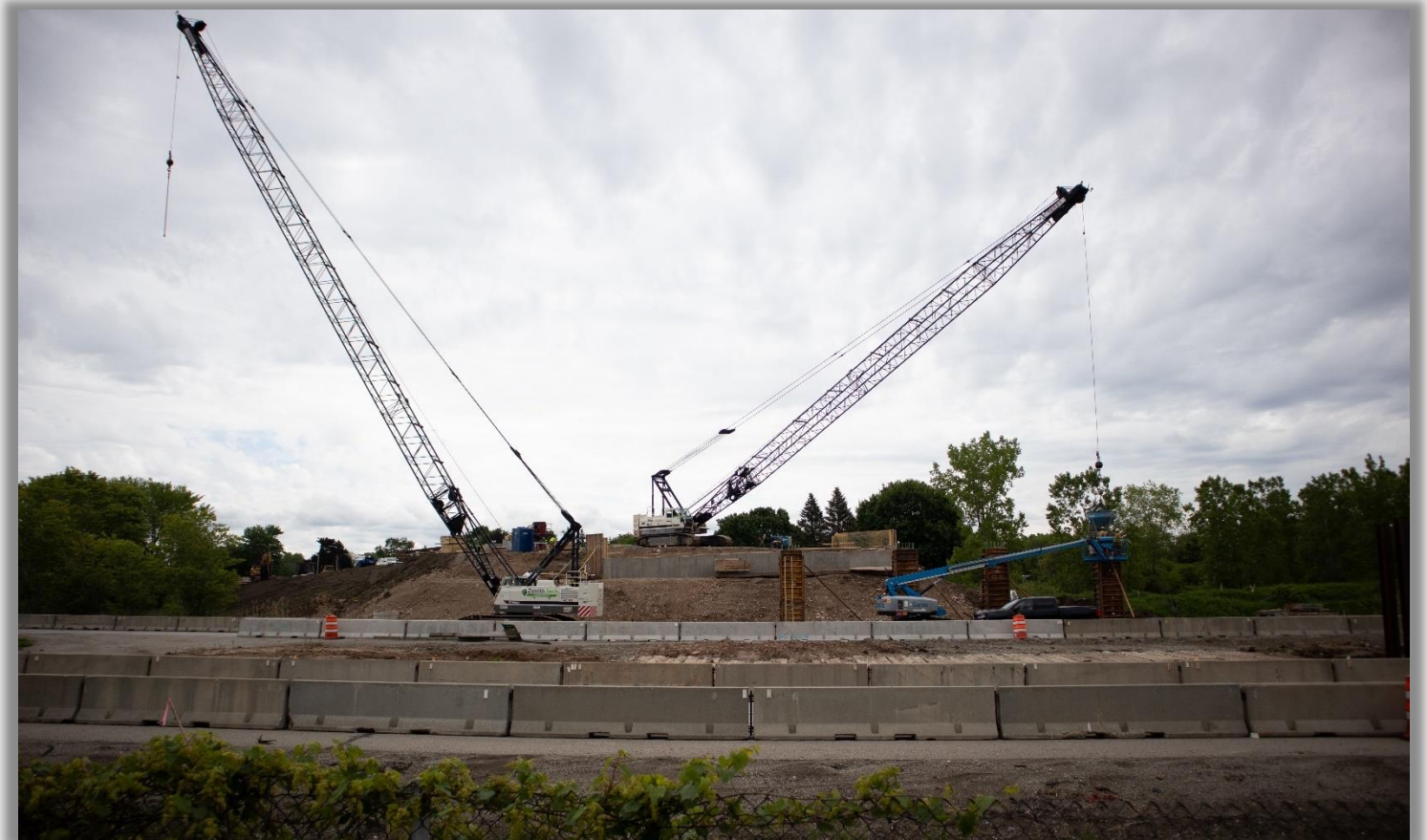
Photo: I-41 expansion, Outagamie County
