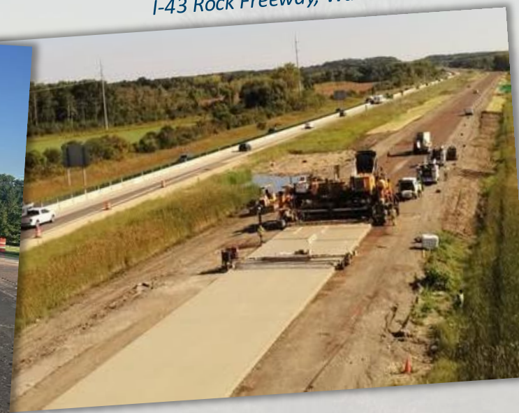
I-43 Rock Freeway, Waukesha County
