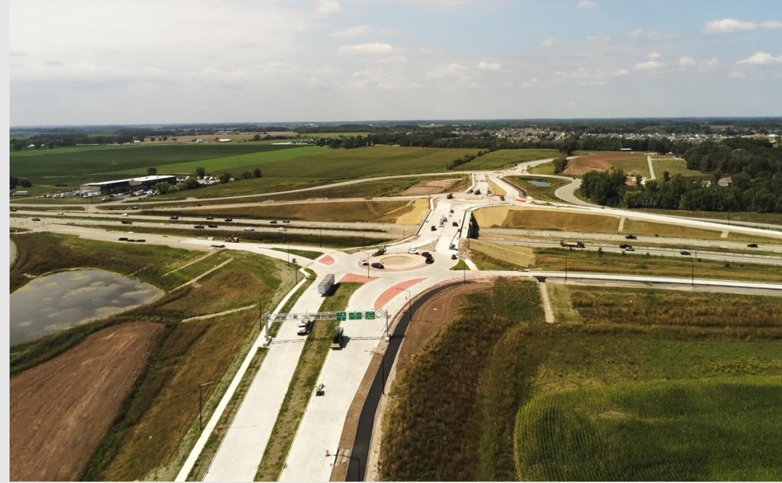
I-41 and Southbridge Road interchange
